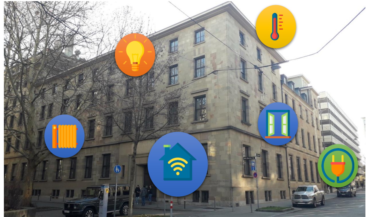
University of Applied Sciences Stuttgart, building 2 (current installation)
