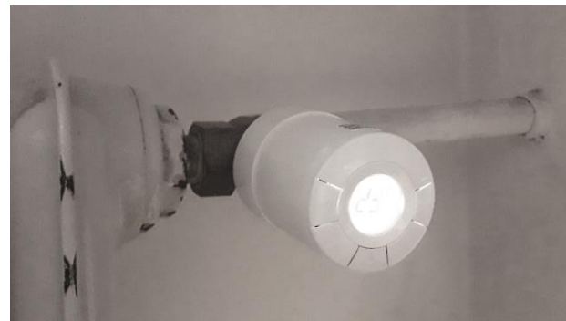
Basic installation: smart switches, thermostats, and multi-sensors in lecture rooms at HFT
